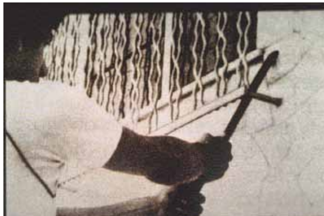
Figure 6: A good steel grille shall not be fastened on the wall, but in direct contact with the window.
