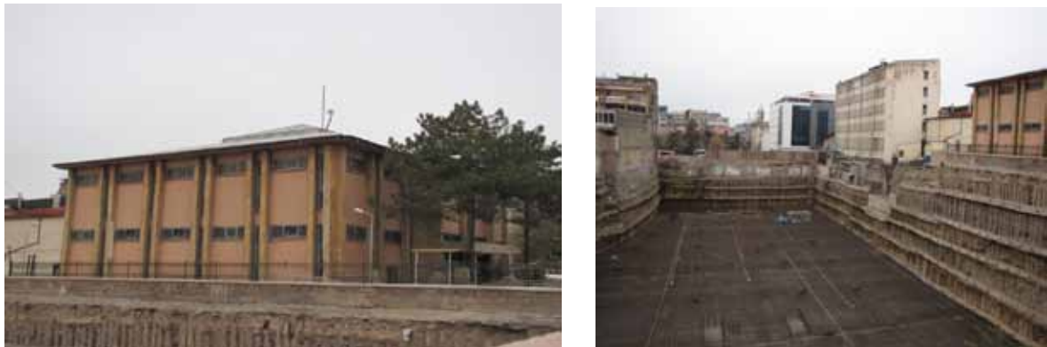
Figure 4: Van Museum and its close environment that was damaged in Van Earthquake happened in 9 November 2011. Deep foundation excavation taking place next to the museum might have increased the vulnerability of building against seismic motions. As it is seen in this example, risk increasing cases happening in close environment of the building should be observed in risk analysis studies.
