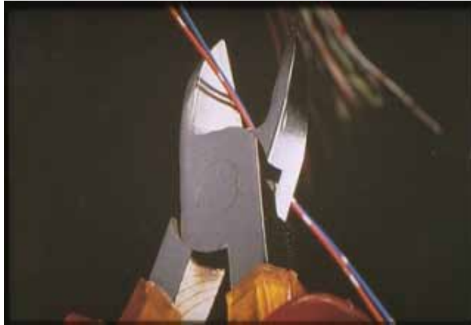
Figure 7: All ingoing and outgoing alarm telephone lines shall be protected against criminal attacks.
