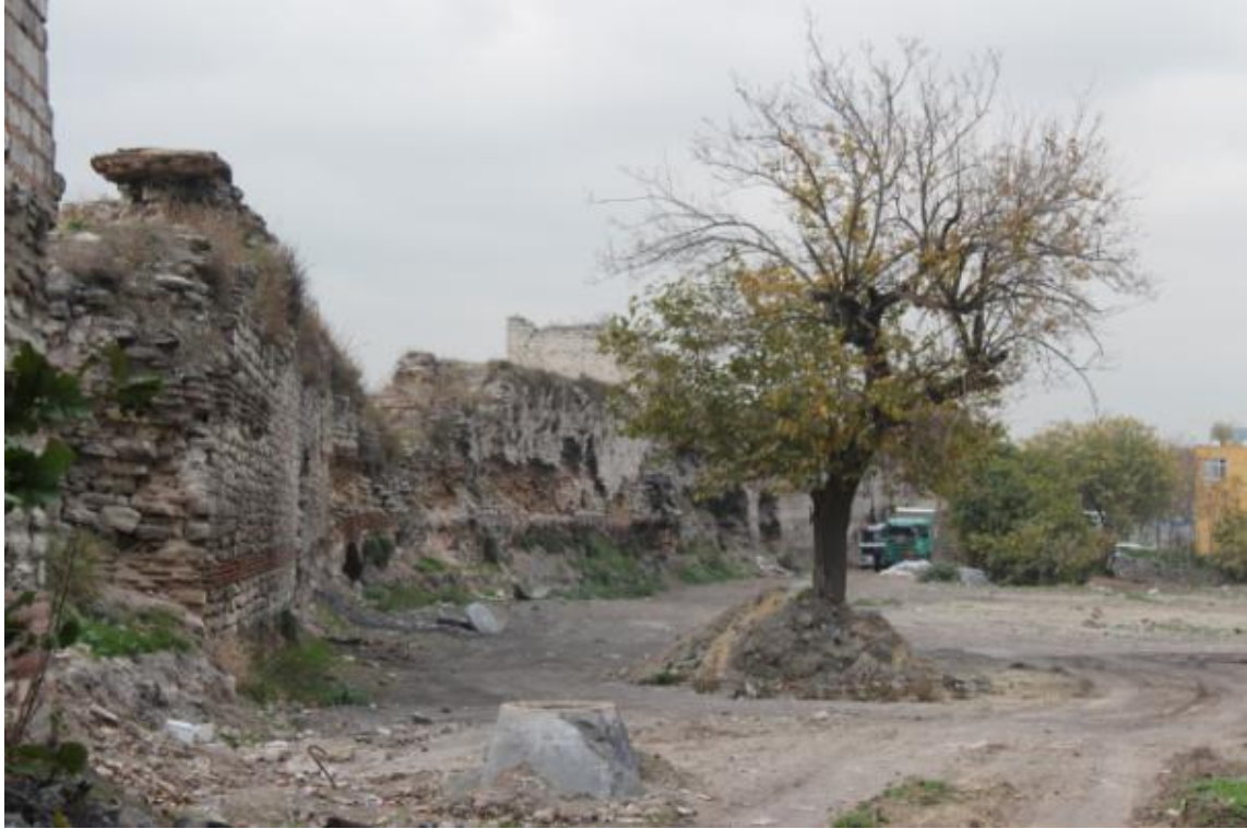
Figure 11 An image showing the destruction of the inner surface of the Inner Walls of the Theodosian Walls, possibly done by bulldozers during the excavation of the bostans (Photo by Figen Kıvılcım Çorakbaş, November 2013).
