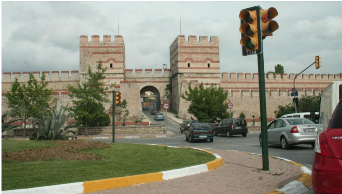
Figure 12 An image showing extensive reconstruction of Belgradkapı Gate (Photo by Figen Kivılcım Çorakbaşı 2013).
