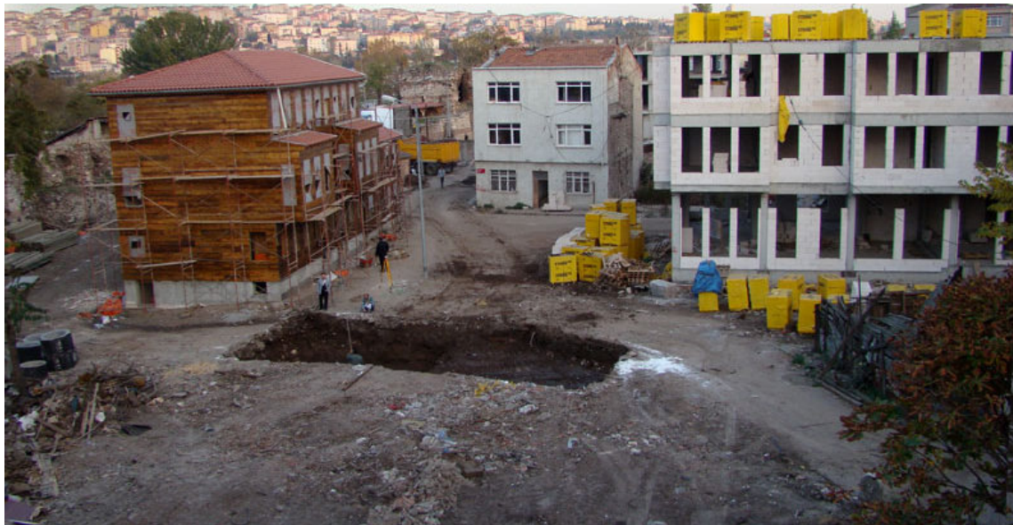
Figure 21 A view of the construction site. Komnenos Walls may be seen on the left.
