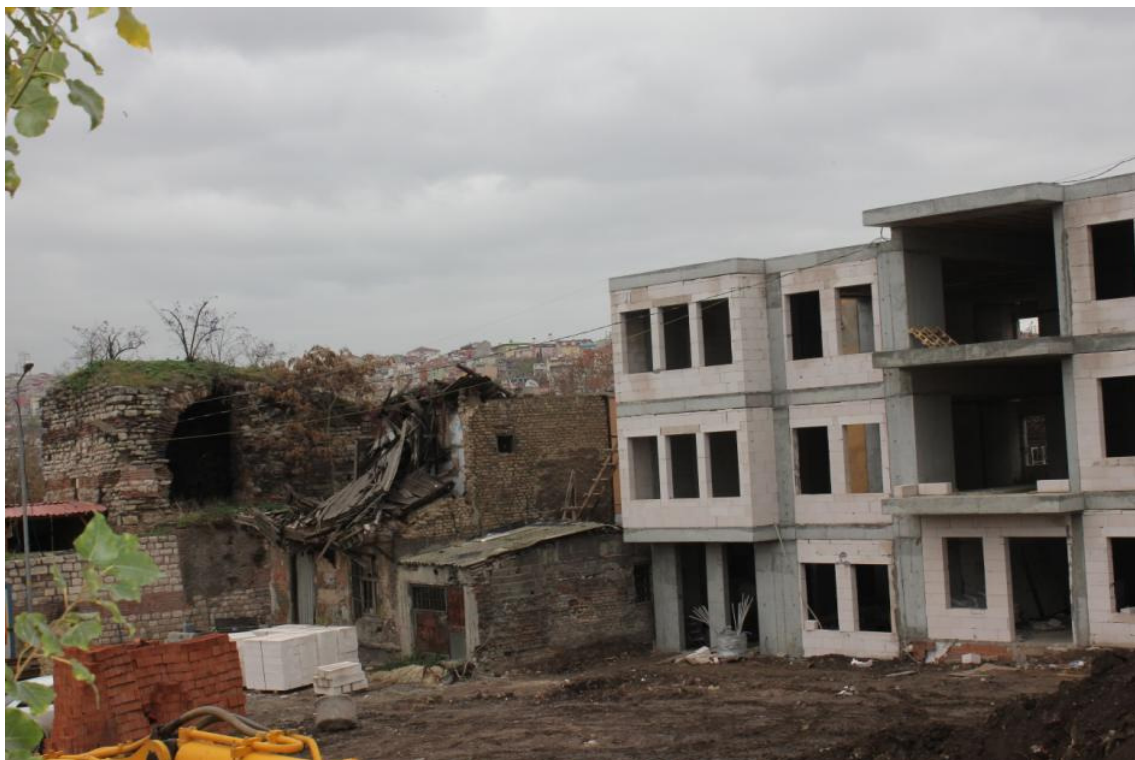
Figure 22 Another view of the construction site. A part of the Komnenos Walls may be seen on the left.
