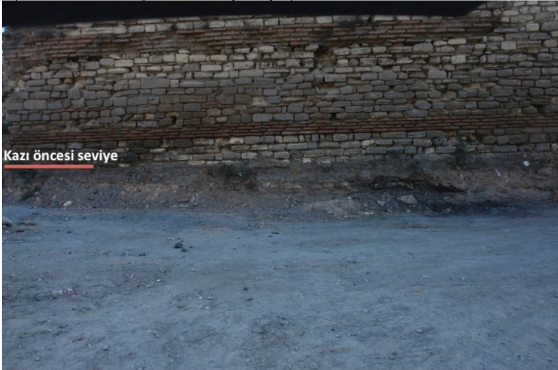
Figure 10 An image showing the difference in ground level line after the excavation (Istanbul branch of Archaeologists' Association, "Yedikule- Belgrad Kapı Arasında Kara Surları İç Koruma Rekreasyon Projesi").
