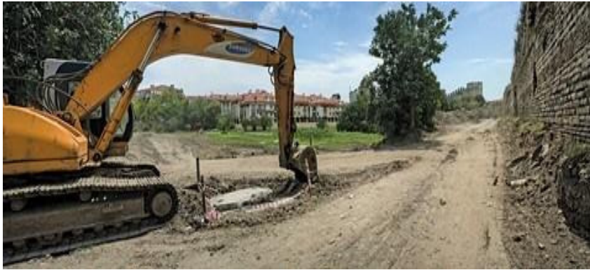
Figure 7 Bulldozer at work in Yedikule. Yedikule Villas may be seen on the background (Photo by Ali Taptık, July 2013).
